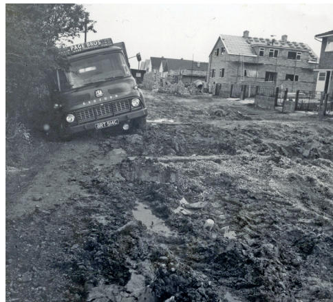
It's 1964 and a lorry sinks up to its axle whilst delivering to the building of Slade Road properties.
