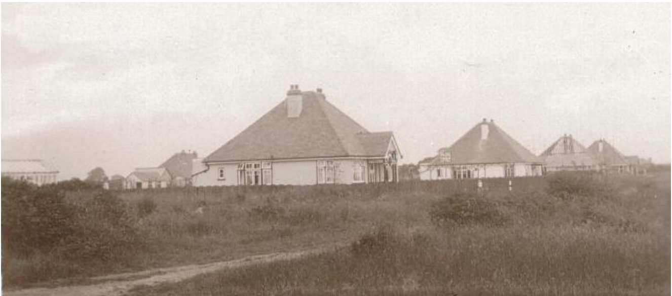
KINGS VIEW ESTATE LITTLE HOLLAND - 1920's THE BUILDING OF BUNGALOWS IN MADEIRA ROAD STARTS TO SHAPE THE IDENTITY OF LITTLE HOLLAND.
