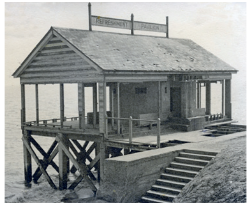
Three years after the end of the Second World War and the now derelict York Road refreshment kiosk still houses a concrete pillbox built during the conflict.
