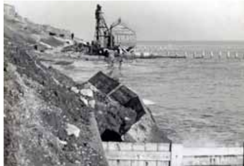
The collapse of a private sea wall, whilst a piling rig gets to work near a derelict cafe.
