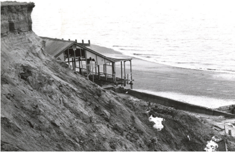
Fiddle Fish Cafe could only be demolished.
