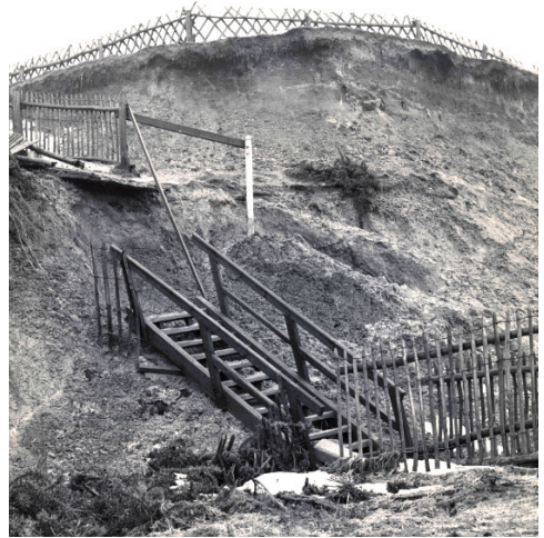
Access to the beach and huts at York Road, following wartime cliff erosion, was no longer possible.
