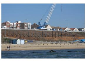
method. Once this has been completed then the buried concrete panels will be installed. When finished the top of this king-post retaining wall will be at cliff level and unnoticeable. Sheet piling behind the C section beach huts will start week commencing 22 October.
